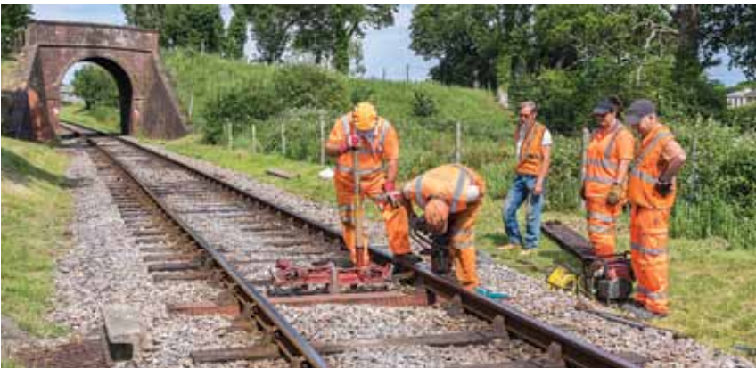
The July working party undertaking sleeper replacement near Deacons Lane bridge. John Faulkner
