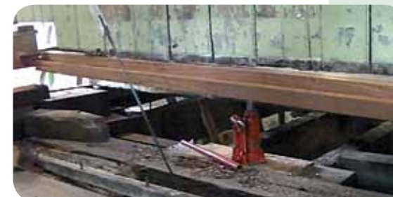
2 May 2019: The new cross-member in process of being fitted. Derek Atkins
