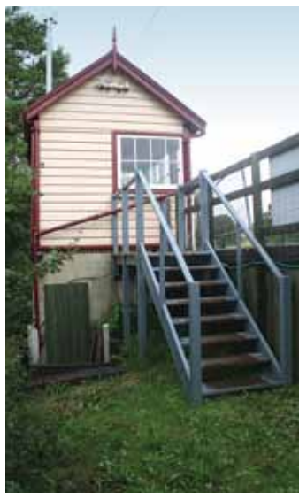
The new staircase at the side of Wootton signal box which gives access to the locking room. Simon Futcher
