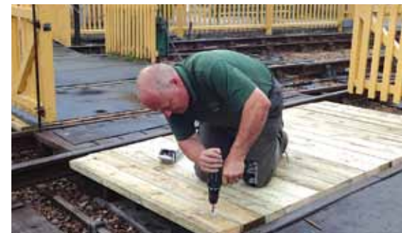
Tim Lee replacing the foot crossing timbers at Havenstreet.
