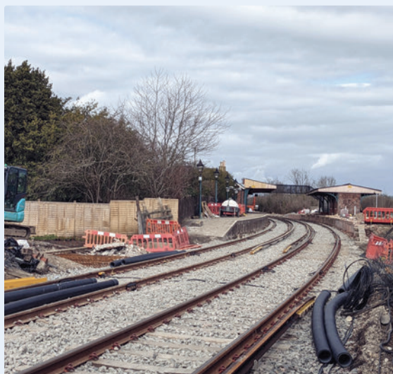
Above: The new curved right-hand point at the London end of Brading station, giving access to the Down Loop (to the left) and the bi-directional Up line, seen on 6 March 2021.
