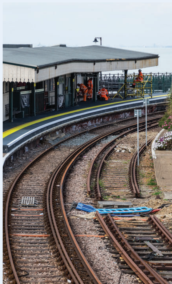
Below: A length of track has been removed from the former Down line at Ryde Esplanade. The gap has been created to facilitate the temporary installation of a signal. The line will be reinstated when a purpose-built cantilevered gantry has been procured. The photograph, taken on 14 May, also shows the Mountbridge platform system in place.
