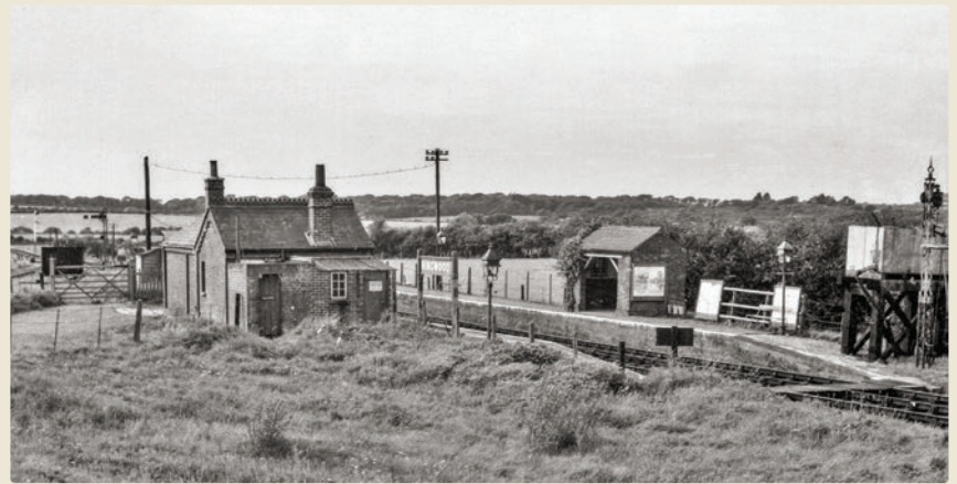
Above: This view was taken from the south side of the ramp of the road overbridge and shows several interesting features; a part of the rear of the station building, the Up waiting shelter and the water tank. [L NWD 007]
