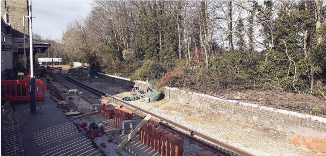
Left: By 11 April track, complete with conductor rail and buffer stop, had been relaid into Shanklin station, although work to complete the retaining wall continues. Andy Merritt
