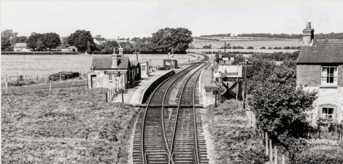
Left: The view from the road overbridge looking towards Freshwater and taken prior to 1936, as witness the loop of original length, but post-relaying with bullhead track and the renewal of the signals with LSWR pattern lower quadrant types. [J Moss L NWD 012]
