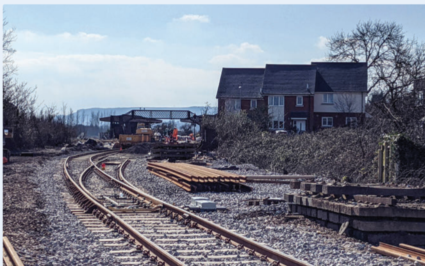
Above: The new curved right-hand point at the London end of Brading station, giving access to the Down Loop (to the left) and the bi-directional Up line, seen on 6 March 2021.
