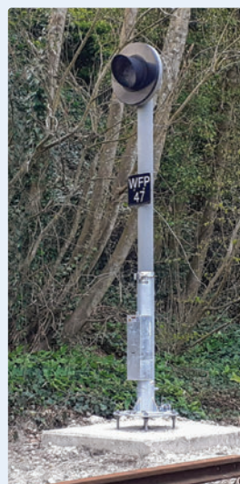
Left: The new Dorman signal WFP47 on the northbound approach to Brading. Traditionalists would probably refer to this as the Brading Up Home signal.
