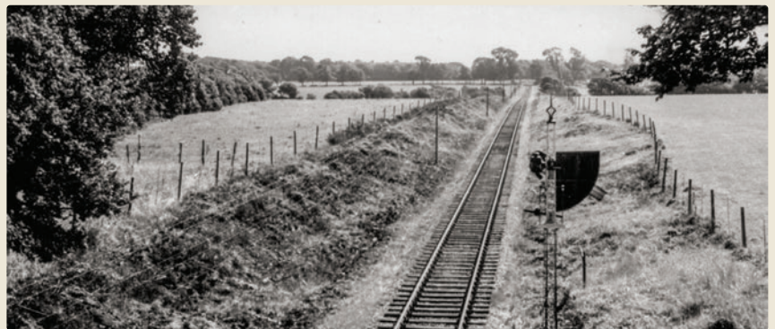
Below: Looking east from the road overbridge towards Newport, the Down Home signal has a sighting board attached to the post to make the arm more visible. Again, the rural location of Ningwood station is very evident. [J Moss L NWD 001]
